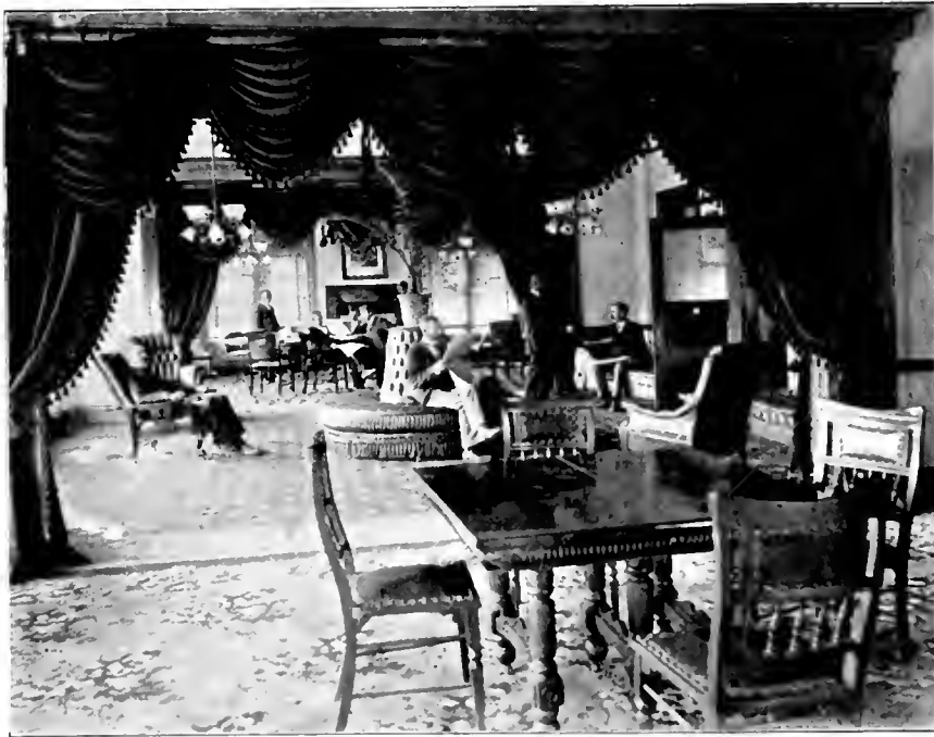
INTERIOR VIEW PARLOR AND DINING ROOM, CAPITAL CLUB. FRANK P. MILBURN Architect Kilough, N. C.
