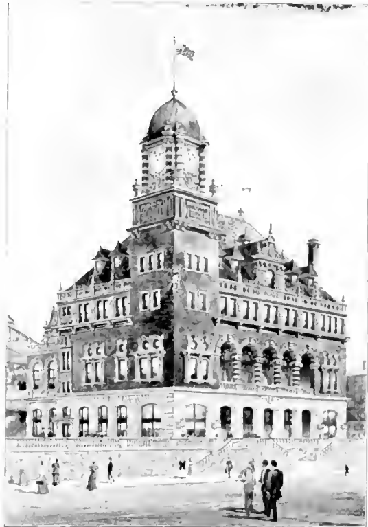
C. & O. -S. A. L. UNION STATION, RICHMOND, VA. HEATED AND LIGHTED BY SMITH-COURTNEY CO.
