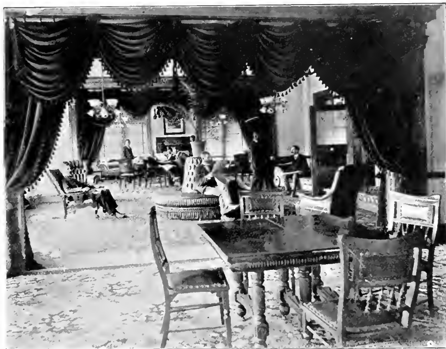
INTERIOR VIEW PARLOR AND DINING ROOM, CAPITAL CLUB. FRANK P. MILBURN, Raleigh, N. C. Architect.
