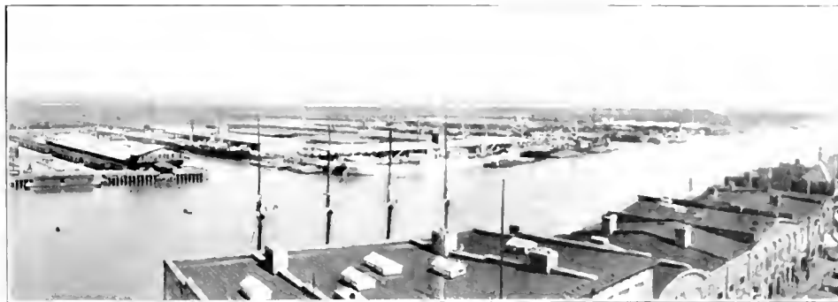
SEABOARD AIR LINE TERMINALS, SAVANNAH, GA.
