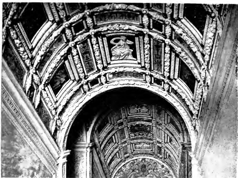
Photo] No. 195. Vault Treatment. Ducal Palace, Venice. Sansovino. [A. Invernizzi]
