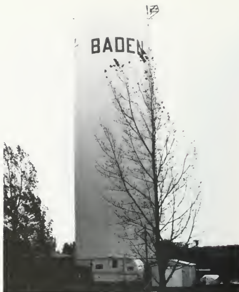
Photo 5-10 Standpipe after insulation (BADEN)
