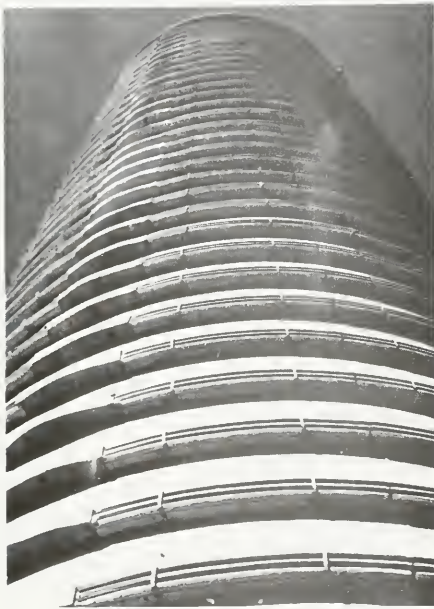
Photo 5-15 External post tensioning (GLENCOE)
