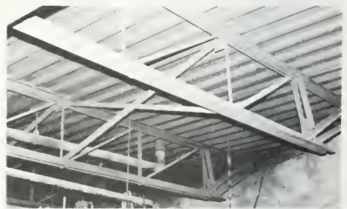
Photo 6-9 Completed roof repair (HESPELER)
