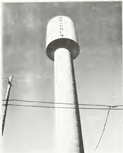
Photo 5-26 Completed rehabilitation of tank. (BRIGDEN)
