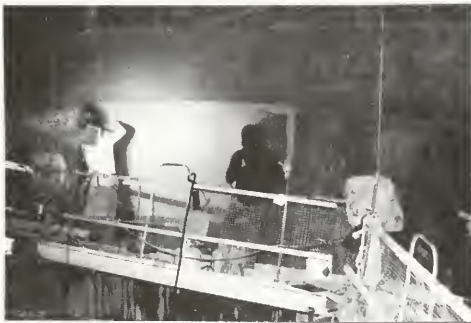
Photo 5-2 Surfacing tank wall prior to application of coating. (HESPELER)
