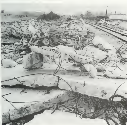
Photo 1-1 Collapsed tank (DUNNVILLE)
