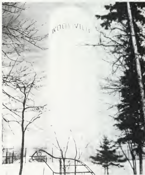
Photo 5-11 Standpipe after insulation (WOODVILLE)
