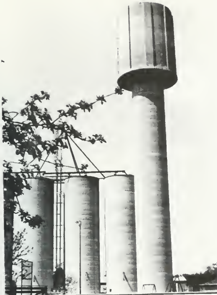
Photo 5-24 Tank after leakproofing and before insulation.(BRIGDEN)
