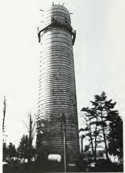
Photo 5-6 Installation of external post-tensioning tendons. (ALVINSTON)
