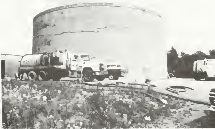
Photo 2-17 Typical cracks and leachate stains occurring at a prestressed ground tank (VAL CARON)
