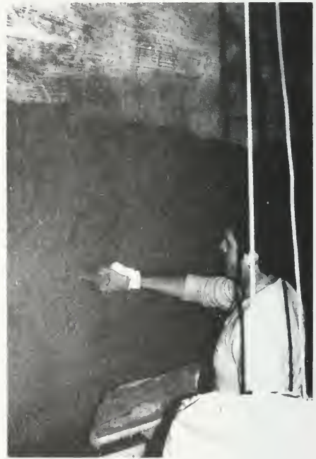
Photo 5-3 Trowelling latex modified mortar. (HESPELER)
