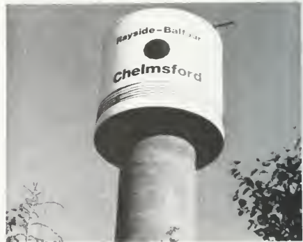
Photo 5-23 Completed repair. Note external tensioning at base of tank. (CHELMSFORD)
