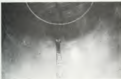
Photo 5-18 Internal maintenance inspection of liner paint system after one year in service (BRECHIN)
