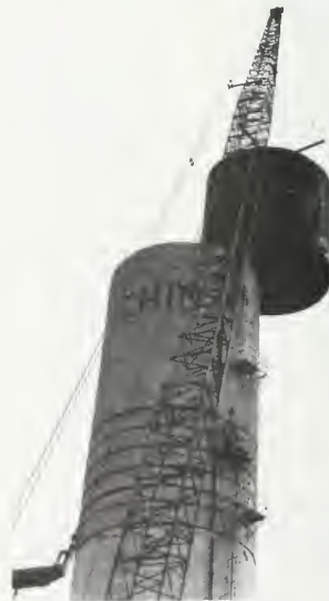
Photo 5-16 Steel liner being installed. Note external post-tensioning (BRECHIN)
