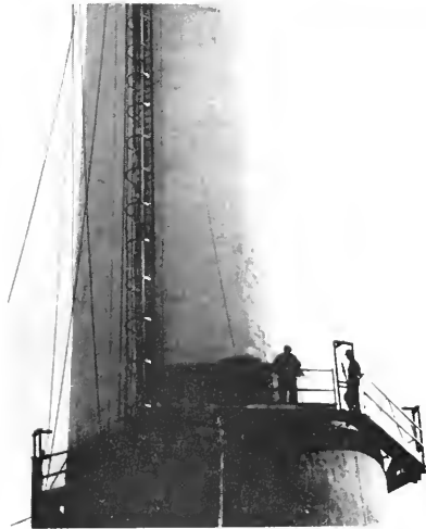
Photo 5-14 Applying coat of MMA to exterior of standpipe (BADEN)
