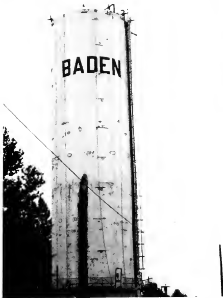
Photo 5-9 Standpipe prior to repair (BADEN)
