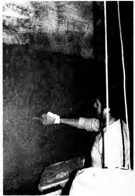
Photo 5-3 Trowelling latex modified mortar. (HESPELER)
