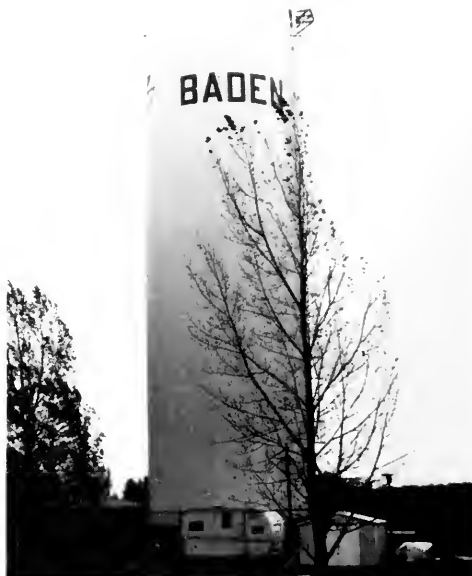
Photo 5-10 Standpipe after insulation (BADEN)
