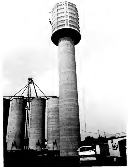
Photo 5-25 Steel support system for insulation and cladding. (BRIGDEN)
