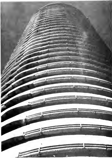
Photo 5-15 External post tensioning (GLENCOE)
