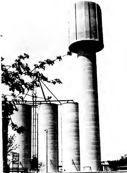
Photo 5-24 Tank after leakproofing and before insulation.(BRIGDEN)
