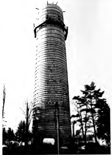
Photo 5-6 Installation of external post-tensioning tendons. (ALVINSTON)
