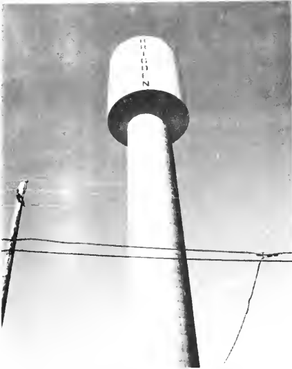
Photo 5-26 Completed rehabilitation of tank. (BRIGDEN)
