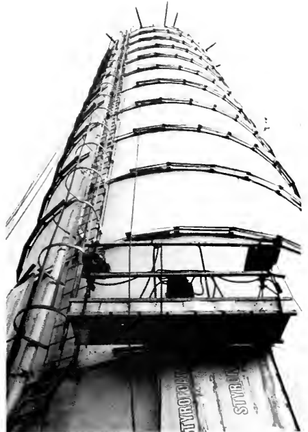
Photo 5-8 Ring support structure for insulation and cladding. (BADEN)
