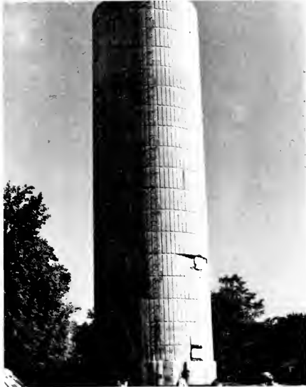
Photo 1-2 Tank implosion. (SOUTHAMPTON)
