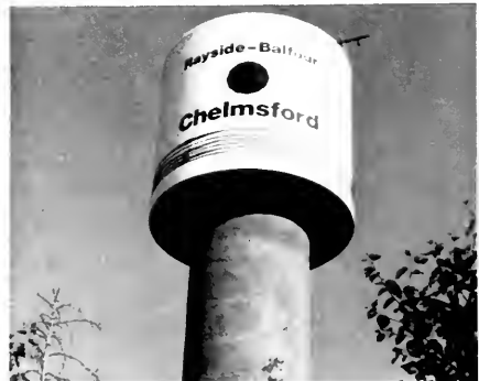
Photo 5-23 Completed repair. Note external tensioning at base of tank. (CHELMSFORD)
