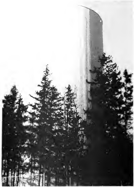
Photo 5-13 Standpipe after insulation (HESPELER)
