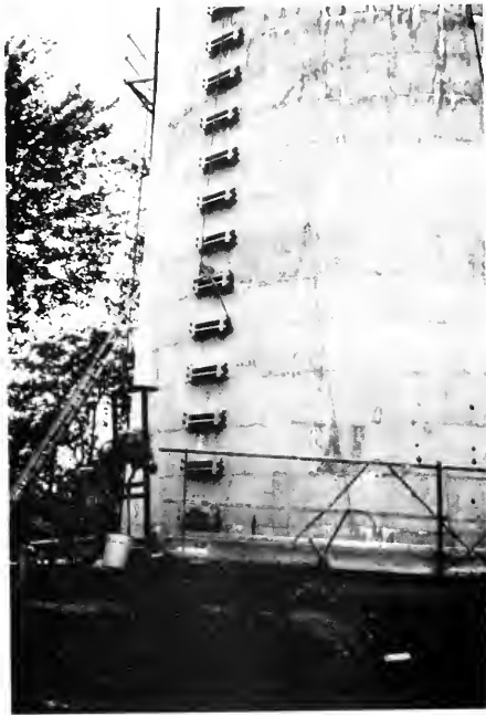
Photo 5-5 Installation of post-tensioning anchors. Note leaks at construction joints. (ALVINSTON)
