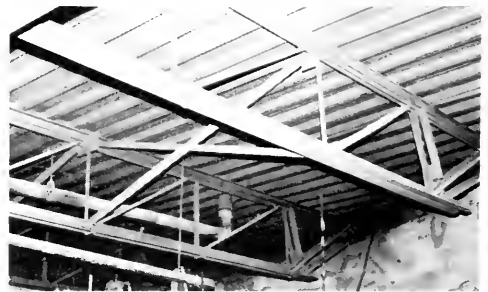
Photo 6-9 Completed roof repair (HESPELER)
