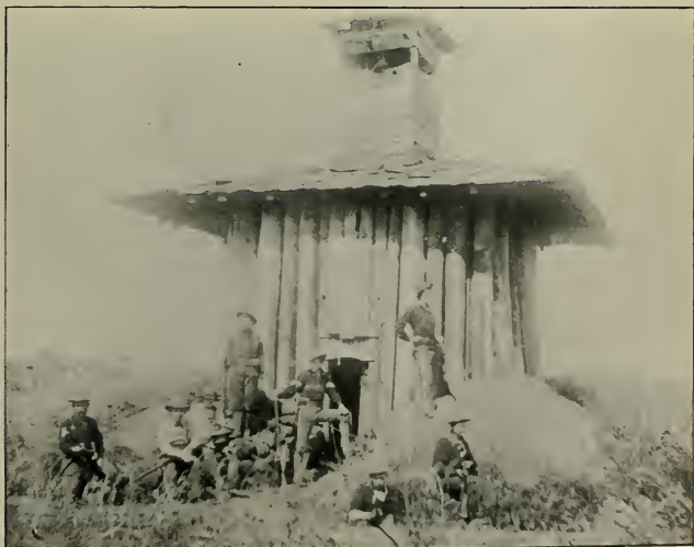
A Blockhouse built of Palmetto Logs, Rodrigo.
