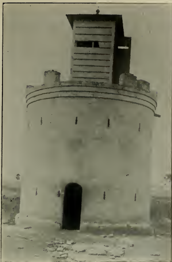
A Masonry Blockhouse at Rodrigo.
