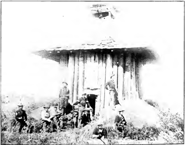
A Blockhouse built of Palmetto Logs, Rodrigo.
