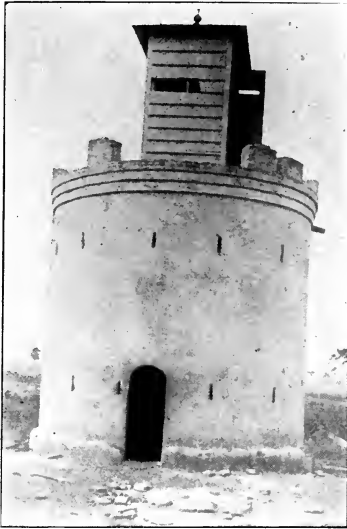
A Masonry Blockhouse at Rodrigo.
