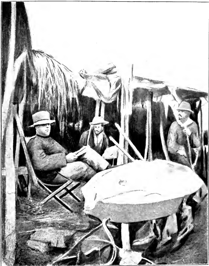
Maj. Wm. G. Latimer, Thirty-fourth M. V. I., in his Headquarters at Sevilla, Cuba, July 14th, 1898, in Command of Six Hundred Men from the Regiment Engaged in Road Building and Keeping it Open Between the Army in Front of Santiago, and the Base at Siboney.
