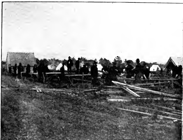
Constructing Tent Floors in Camp at Amaro under Major Harrah's direction.
