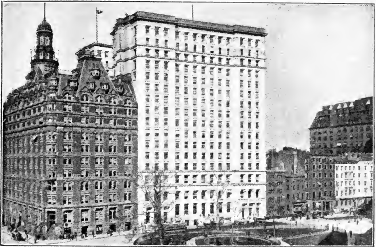
Das Bowling-Green-Building in New York.
