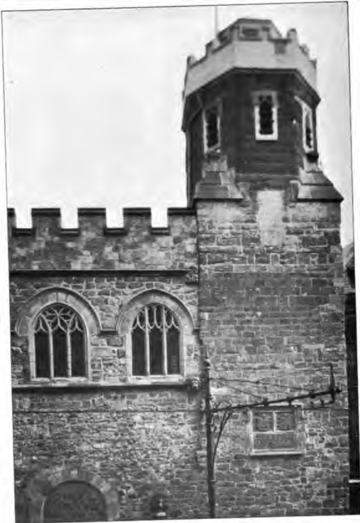
Tower of St. Petrock's.
