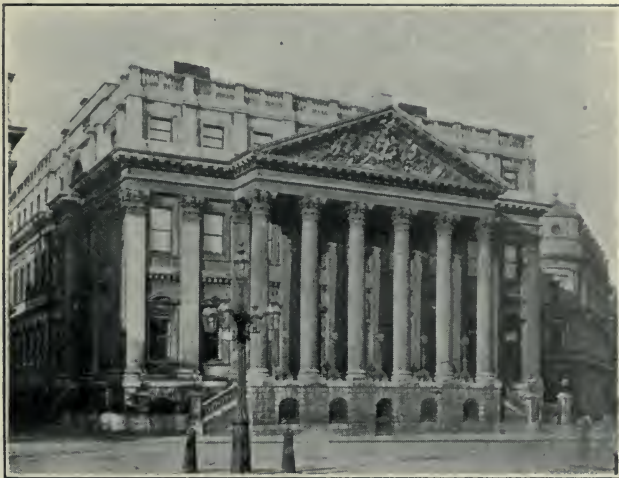
Fig. 7. Mansion House, London.
