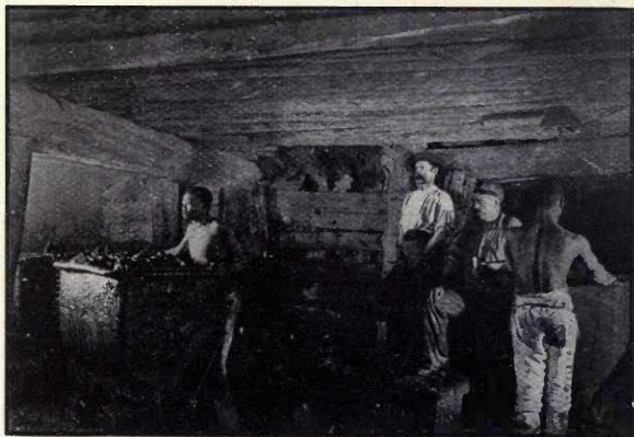
FIG. 7. DE BEERS MINE. UNDERGROUND WORKINGS.
