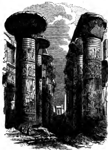
AVENUE IN THE GREAT HALL OF COLUMNS AT CARNAC, THEBES.
