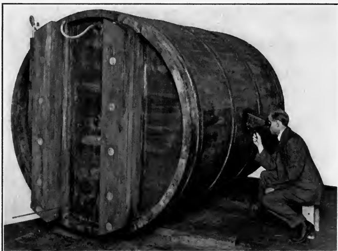
FIG. 96.—Cask for the study of the variation of spark-over and corona voltages with air pressure.
