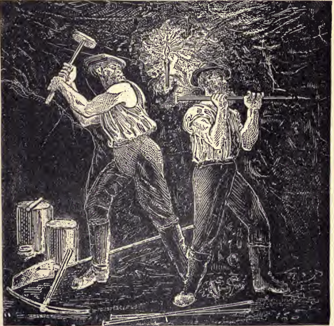
HAND-DRILLING IN THE MINE.
