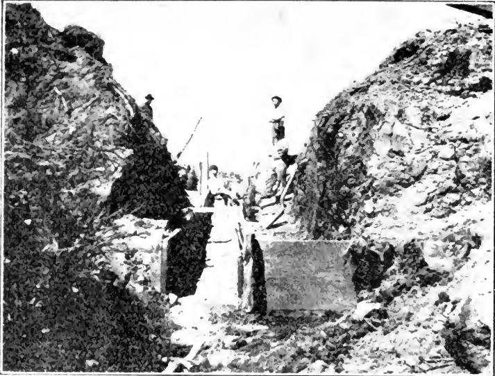
SIMON GEORGE REBUILDING WORTHLESS FLUME PLACED BY INDIAN SERVICE ACROSS WAPATO CANAL
