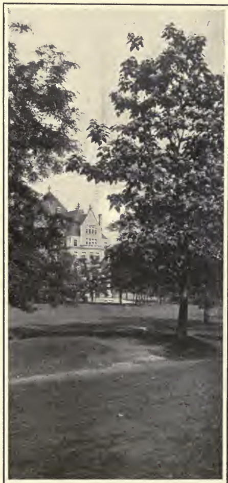
LOOKING ACROSS THE QUADRANGLE OF THE UNIVERSITY OF CHICAGO TOWARD GREEN HALL
