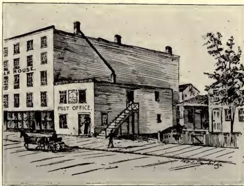
THE SECOND BUILDING WHERE THE CHICAGO POST OFFICE WAS KEPT.
