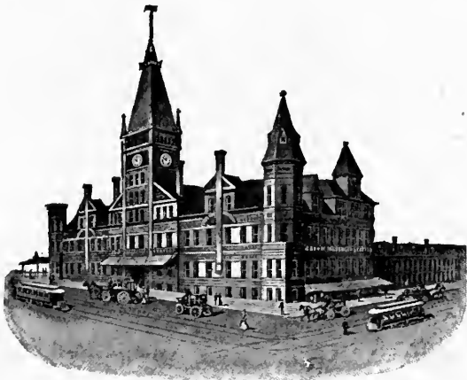
WELLS STREET DEPOT, CHICAGO & NORTH WESTERN R' Y
