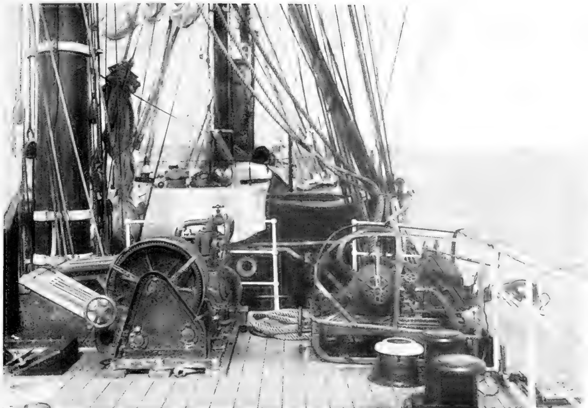
Fig. 1. R.R.S. 'Discovery'. View on forecastle head, looking aft, showing Lucas sounding machine on right, and deep-water hydrological machine on left.
