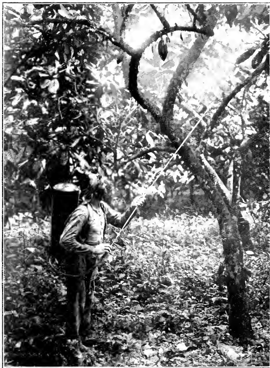
Fig. 29 COMPRESSED AIR SPRAYER IN ACTION
