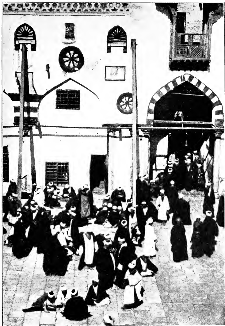
INTERIOR OF MAIN COURT, EL AZHAR UNIVERSITY, CAIRO. Showing the dilapidated condition of the building.
