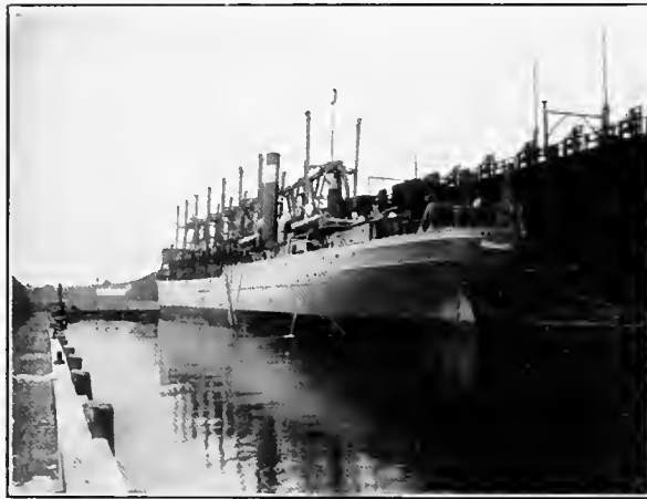
COAL PIER, CURTIS BAY.
