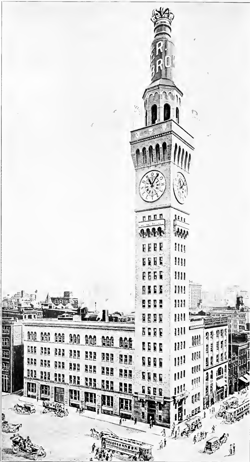
BROMO-SELTZER TOWER. Total height of tower, 357 feet. The Bottle on top, a fac simile of the regular ten-cent Bromo-Seltzer bottle, but about 10,000,000 times larger, is 51 feet high, 20½ feet in diameter, weighs 17 tons, and revolves at the rate of 107 feet per minute. There are 500 electric lights in bottle and crown surmounting it, which can be seen at a distance of 20 miles. The Bromo-Seltzer clock is the largest four dial gravity clock in the world. The dial is 24 feet in diameter. The minute hand is 12 feet 7 inches long, and weighs 175 pounds. The hour hand is 9 feet 8 inches long and weighs 145 pounds. The pendulum is 15 feet long and weighs 45 pounds. The clock is automatically wound by an electric motor every six hours.
