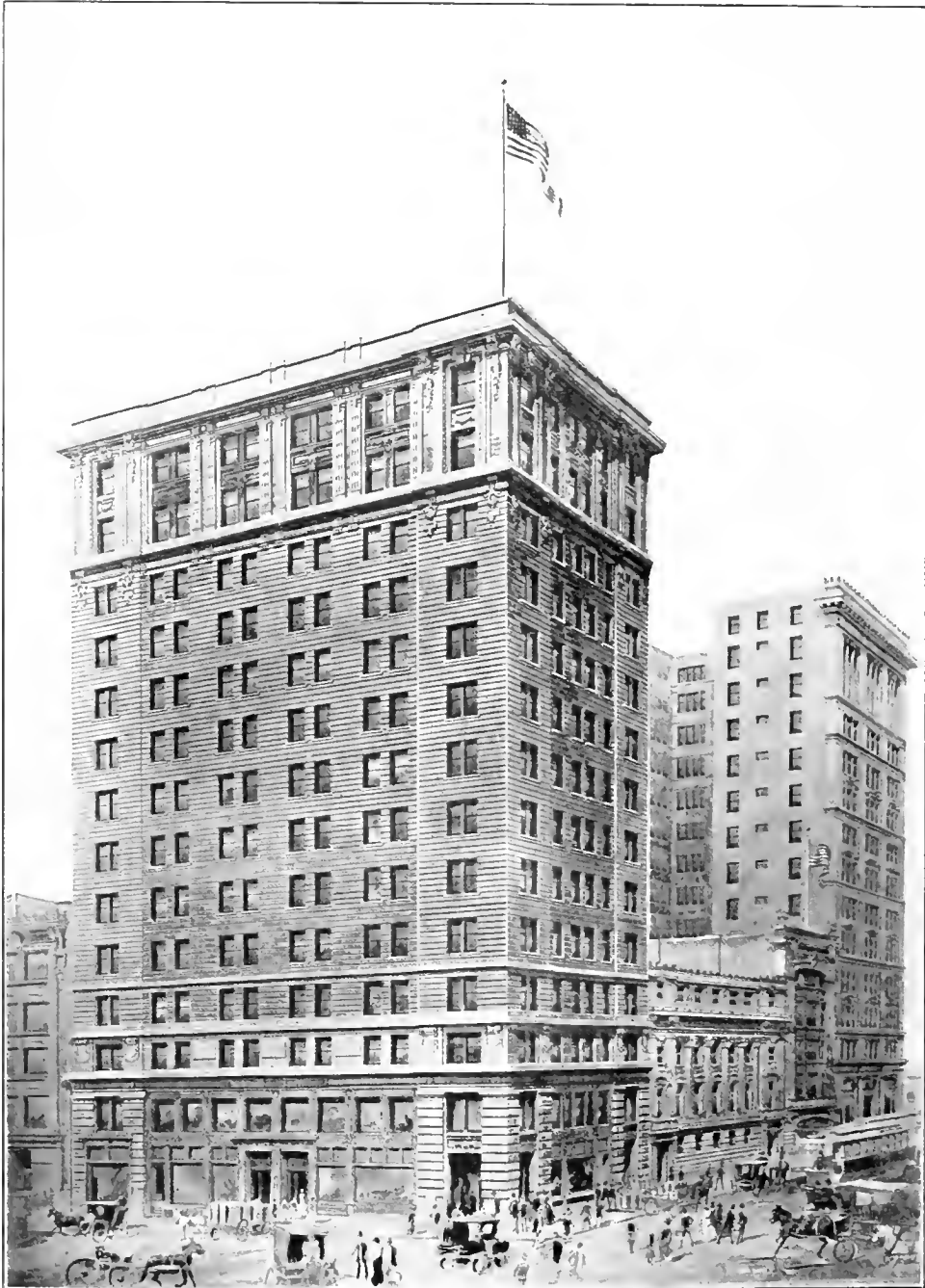
THE AMERICAN BUILDING is one of Baltimore's most imposing skyscrapers. As the home of the oldest newspaper in America it contains one of the best equipped newspaper plants in the whole country, installed and constantly improved in a persistent endeavor to give The American's readers the very best service obtainable. The building stands a substantial proof of The American's faith in Baltimore. It was the first large structure erected after the fire, and the lofty building that rose upon the ashes of the smaller one was an inspiration to Baltimore. We Build is the motto of The American, and it has done full measure of service in promoting the interests of the city and state. The American building represents an investment of over a million dollars, aside from the equipment. It is 16 stories high, houses five sextuple presses with a capacity of 225,000 papers an hour, and 25 linotype machines, in addition to all the necessary machinery which goes to make up a first class newspaper office. The exterior is imposing, the interior artistic in decoration, and the building and plant as a whole testimony to The American's firm faith in the future of the Greater Baltimore.
