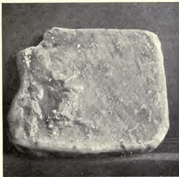
FIG. 683.—Positive Plaster Cast of Electrolytic Pitting on 14-inch Cast-Iron Main.
