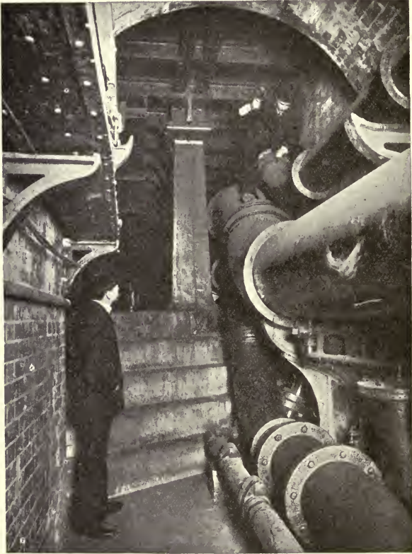
FIG. 188.—Holborn Subway, showing Alteration of Levels.
