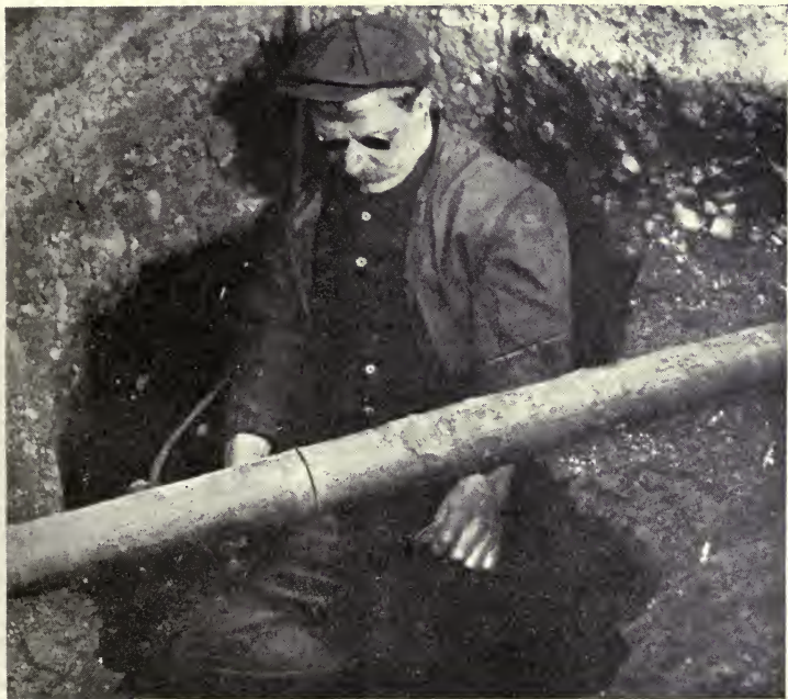
FIG. 70.—Welding Joint in Trench.
