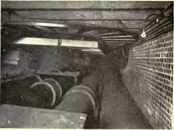
FIG. 190.—Mansion House Subway.
