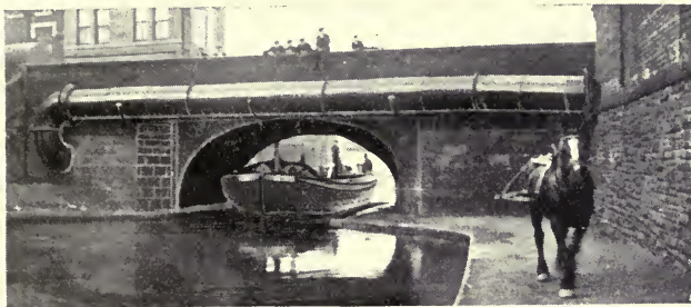
FIG. 54.—Elevation of 36-inch Steel Main over Leeds and Liverpool Canal, New Wortley, Leeds.
