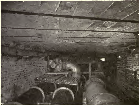
FIG. 191.—Mansion House Subway.
