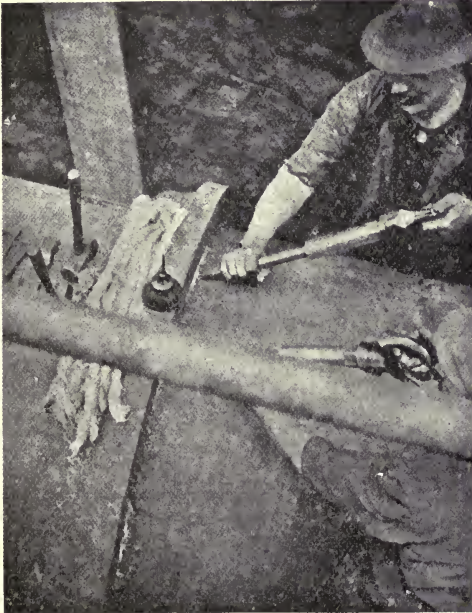
FIG. 100.—Caulker working on 48-inch main.
