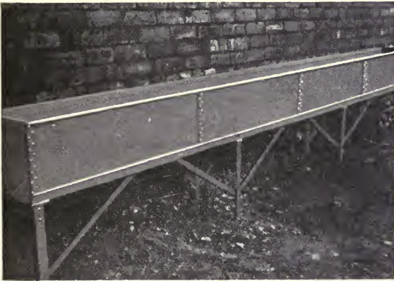
FIG. 199.—Pipe-Dipping Tank.
