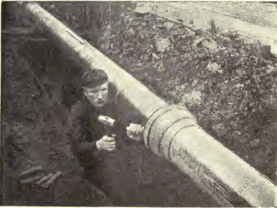
FIG. 135.—Setting Joint Up from Trench.
