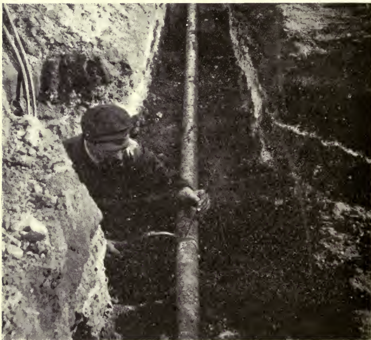
FIG. 69.—Welding Joint in Trench.
