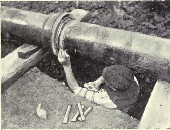
FIG. 134.—Setting Joint Up from Trench.
