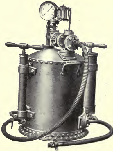
FIG. 142.—Milne's Leak-Testing Machine.
