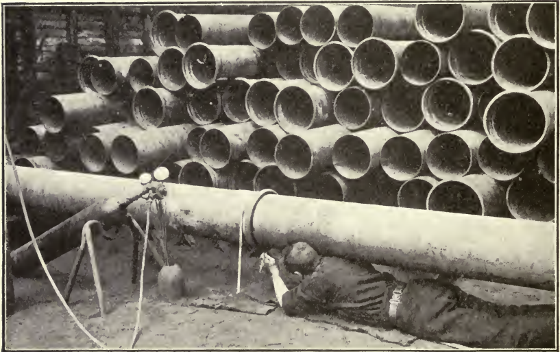
FIG. 72.—Welding Gas Main without turning pipe as done in Trench.
