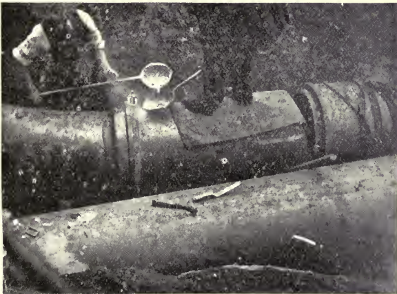
FIG. 91.—Running Large Joint from two Ladles
