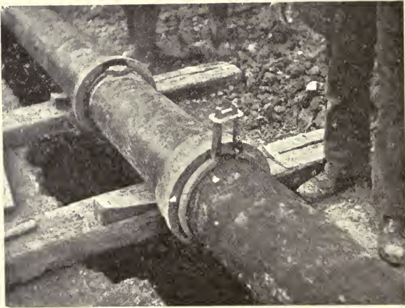
FIG. 89.—Clips Fixed on Pipe.
