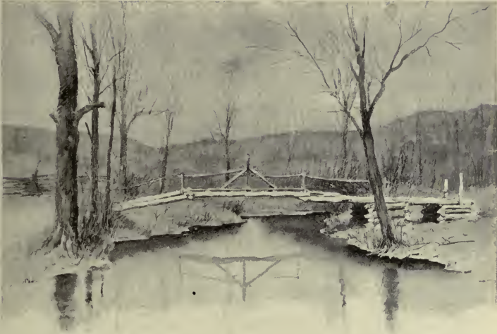
A FOOT-BRIDGE, WEST VIRGINIA
