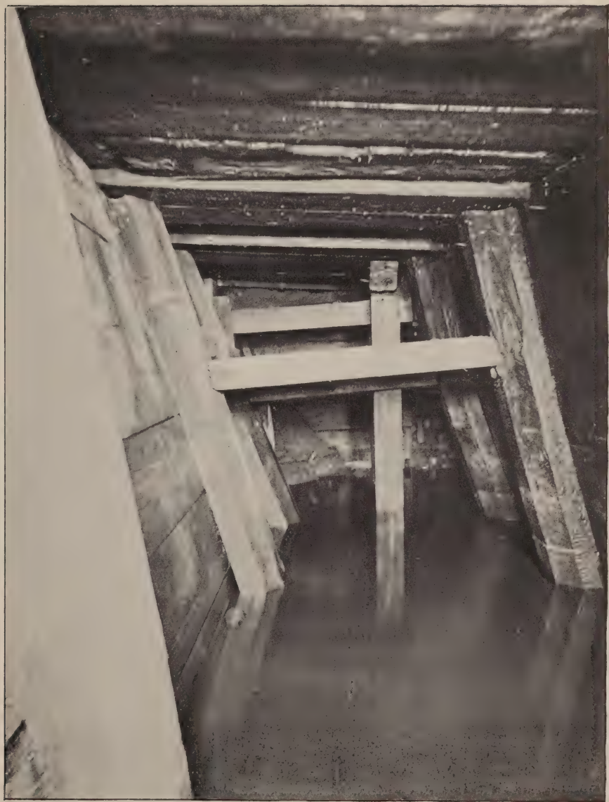
OLD WOODEN SEWER—DOVER STREET.
