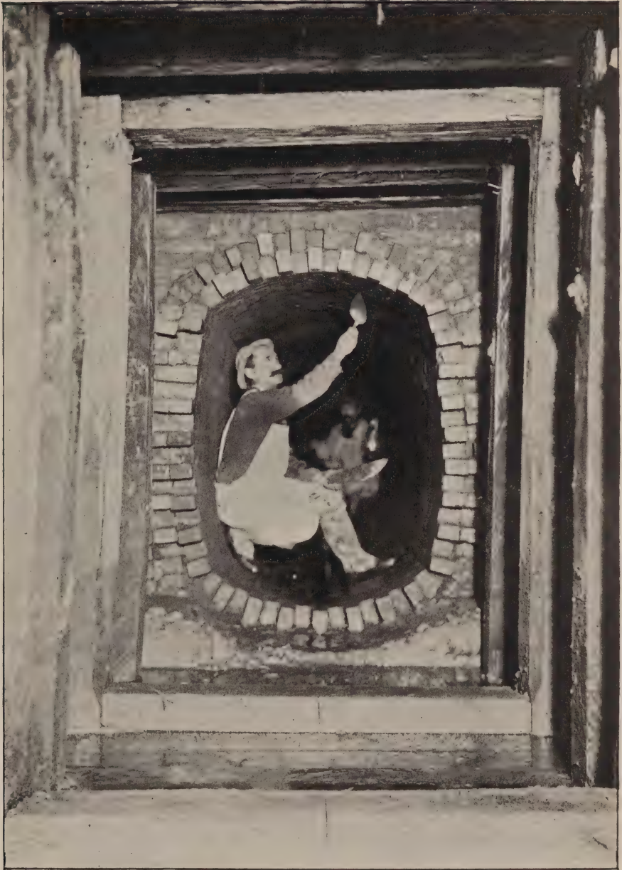
MASONRY CONSTRUCTION WITHIN DOVER-STREET SEWER.
