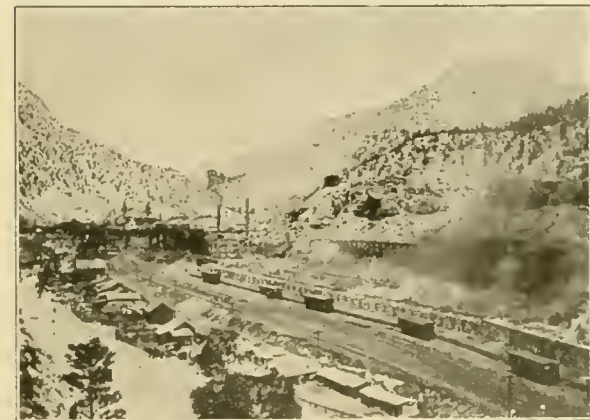
FIG. 10. Coal mines and coke ovens, Castlegate. Coal from this field produces coke which, as an ideal fuel for industrial plants, bids fair to rival the celebrated Connellsville product.
