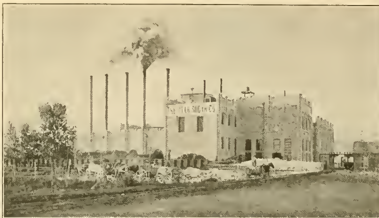
FIG. 71. Beet-sugar factory at Lehi. This was the first sugar factory established in Utah.
