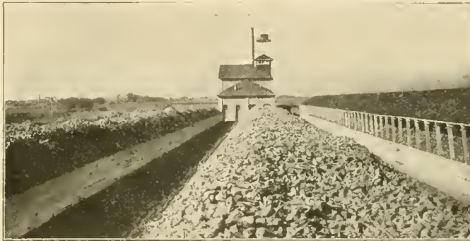
FIG. 50. A sugar-beet crusher, Provo. In the foreground may be seen 7,000 tons of beet root awaiting the crusher. The juice will be pumped to the sugar refinery at Lehi, twenty-five miles away.
