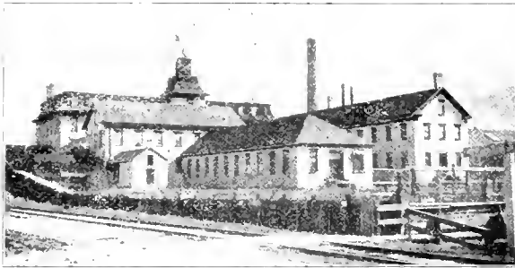
FIG. 46. Woolen mills at Provo. Established by Brigham Young in 1872, they were the first erected west of Chicago, and are now the largest woolen mills west of the Missouri River.
