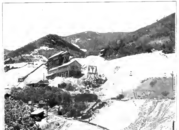
FIG. 41. Head house, Gabriel mine, Bingham Canyon. Notice the aerial tramway for sending the ore to the mill.
