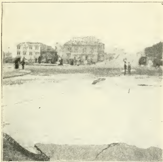
Fissures on Van Ness Avenue, San Francisco, showing the cracked and broken pavement.
