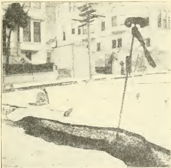
One of the many fissures in San Francisco's streets.
