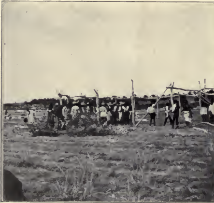
FIG. 44. Erecting the lodge.
