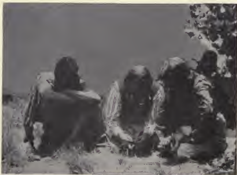
FIG. 28. Filling the sacred pipe.
