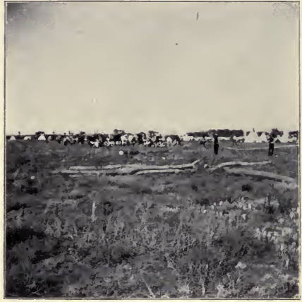
FIG. 43. Preparing the timbers for the lodge.
