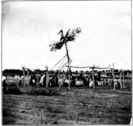
FIG. 54. Raising the center-pole.
