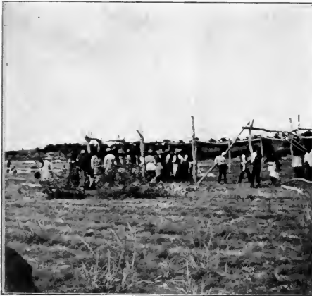
FIG. 44. Erecting the lodge.
