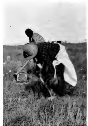
FIG. 46. Digging the hole for the center-pole.
