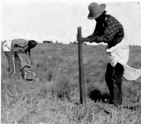
FIG. 46. Digging the hole for the center-pole.
