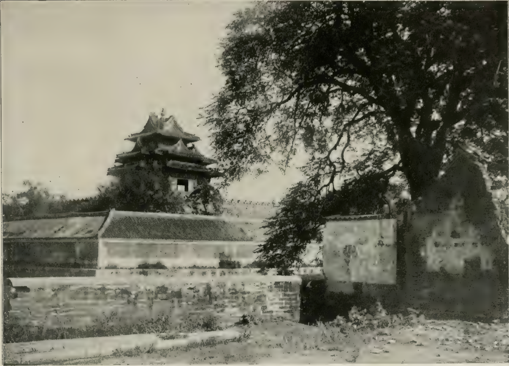
NORTHWEST ANGLE OF THE PURPLE WALL
