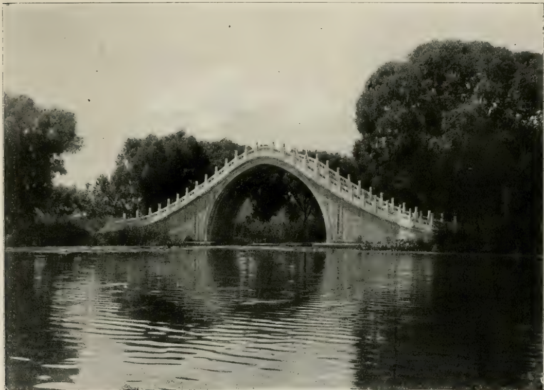
THE MARBLE BRIDGE OF THE SUMMER PALACE
