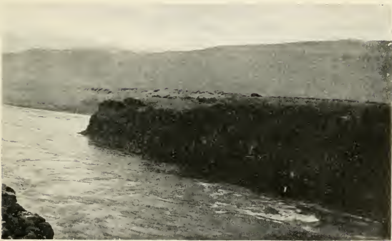
LIFTED DRAWBRIDGE ON CELILO CANAL ( above ) TUMWATER CORGE OF THE GRAND DALLES ( below )
