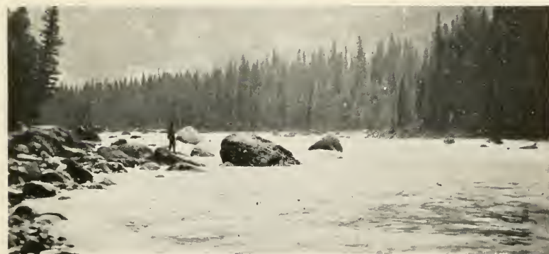
“SHOOTING” THE FIRST BIT OF LINING AT SURPRISE RAPIDS ( above )
