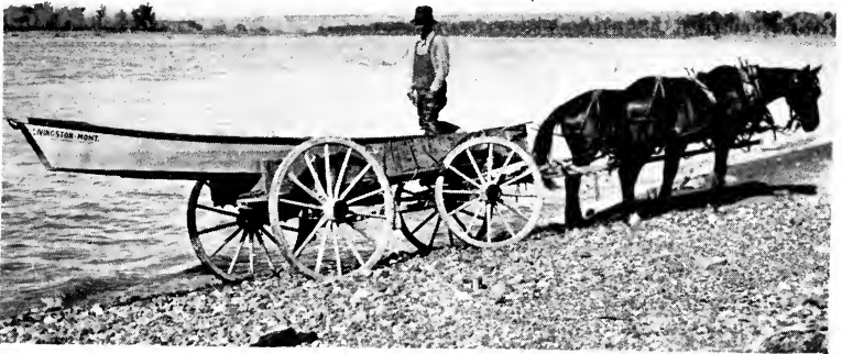
THE DAM ACROSS THE YELLOWSTONE AT INTAKE ( Above ) PORTAGING MY BOAT ROUND THE INTAKE DAM ( Center ) COMPLETING THE PORTAGE ( Below )
