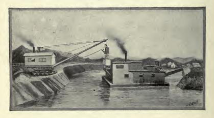
This "Drag Bucket" excavator is mounted on rails and operates ahead of the washing apparatus. It has a long boom (about 100 feet in length) from the outer end of which the bucket is operated by a cable line. The whole apparatus is mounted upon a turn-table and
