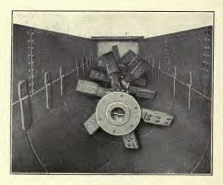
tus that we guarantee to successfully handle both clay and ground containing gravel and clay mixed. For material containing only a small amount of clay, or clay and gravel mixed, we build a large clay disintegrating and washing machine through which all the material passes before reaching the screen and gold saving tables. This machine completely breaks up the clay, which then passes into the
