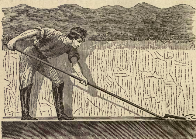
Fig. 30.—POSITION OF WORKMAN AND USE OF FINISHING SCOOP.
