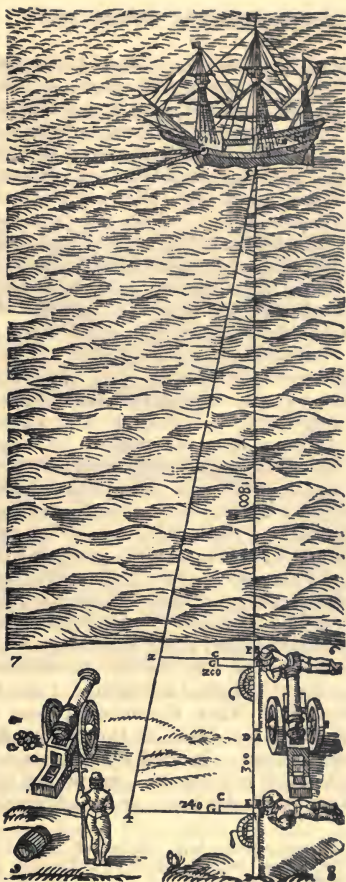
RANGE-FINDING BY MEANS OF THE GUNNER'S 'HALF-CIRCLE' (FROM TARTAGLIA'S 'COLLOQUIES,' 1588)
