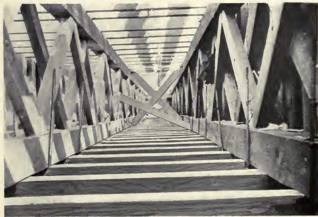
INTERIOR OF HULL SHOWING FRAMING
