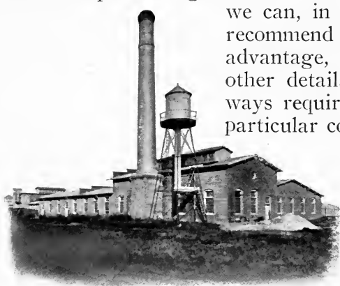
POWER HOUSE—CENTRAL PLANT
