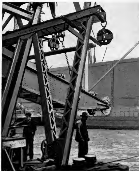
DETAIL OF STEEL GANTRY
