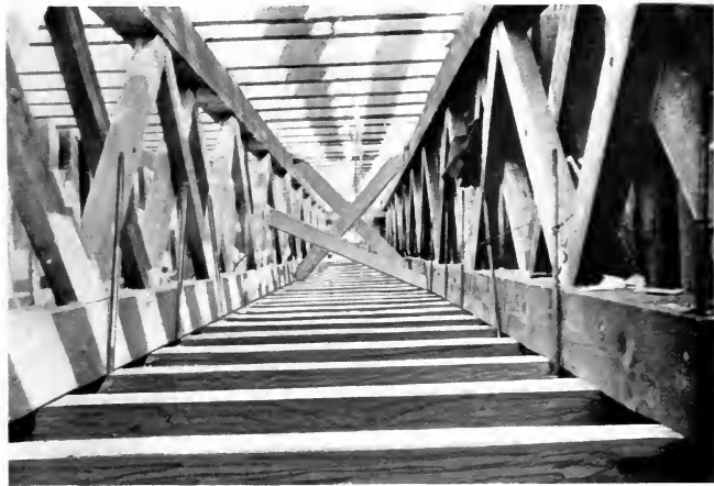
INTERIOR OF HULL SHOWING FRAMING
