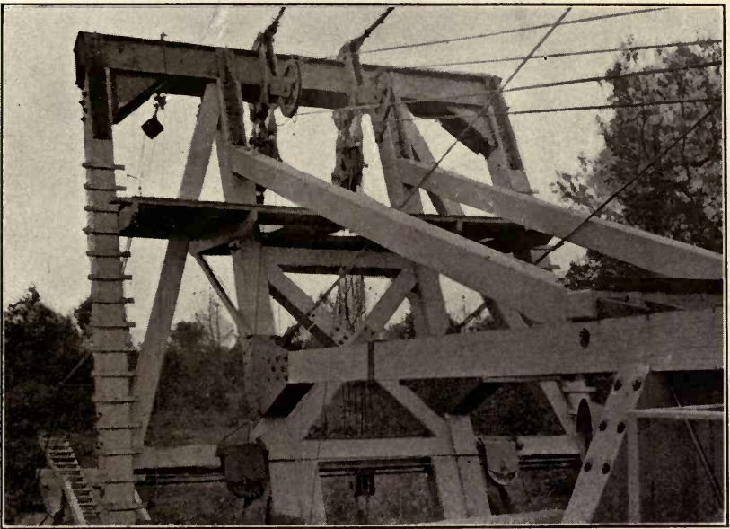
Fig. 21. Forward Gauntree on Boston No. 4 showing Steel Cap and Method of Bracing in Rear.
