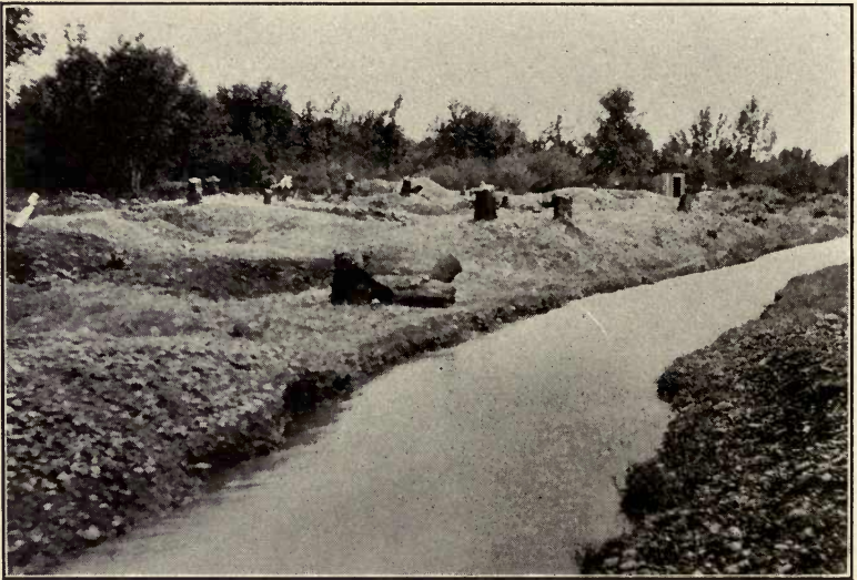
Fig. 50. Removing Stumps along Irrigation Ditch in Front of the Nevada.
