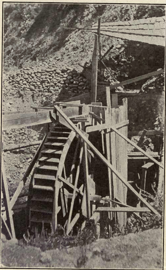
Fig. 97. Old Chinese Workings at Folsom, showing Home-Made Water-Wheel for Chinese Pump.
