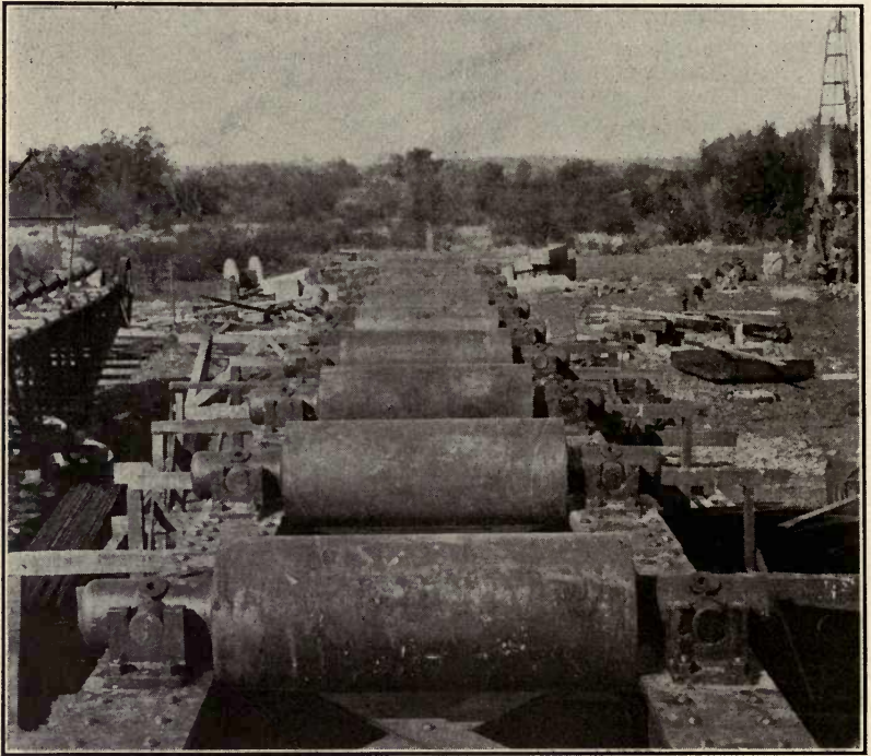
Fig. 24. Rollers on Digging-Ladder, No. 3 Folsom.
