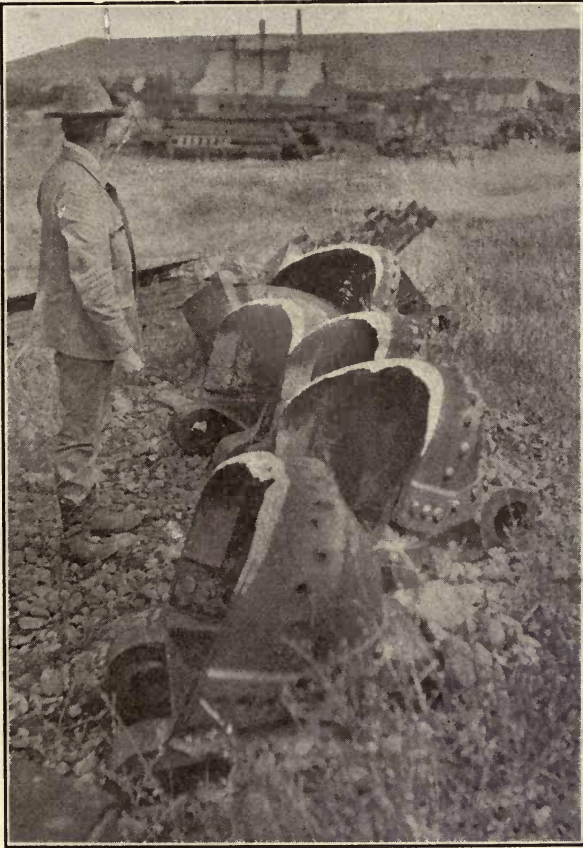
Fig. 91. Showing Wear on Lips of El Oro Buckets.
