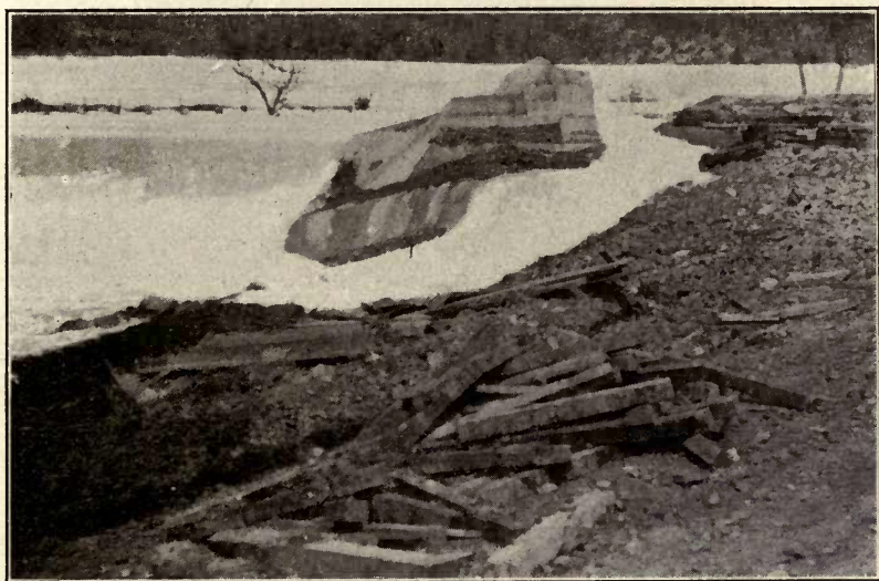
Fig. 6. Spillway of the Barrier Dam on the Upper Yuba.
