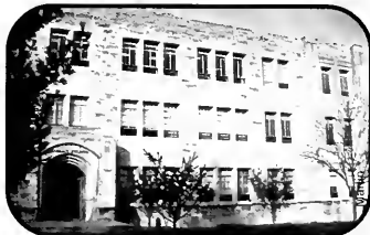
Pharmacy Building Completed in 1951
