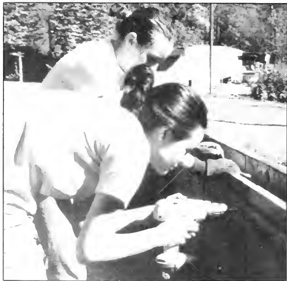
Freshmen Nicole Godfrey (back) and Leah Winkler prepare to pour concrete.
