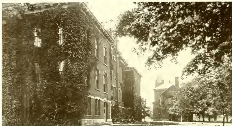
ADMINISTRATION AND SCIENCE BUILDINGS
