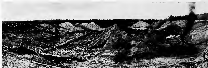
Panorama View of Stadium Under Construction
