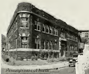
Pennsylvania at North
