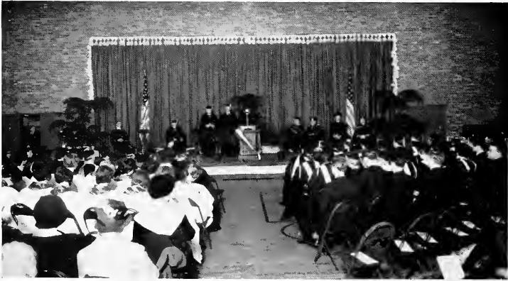
INSTALLATION OF THE COLLEGE OF EDUCATION
