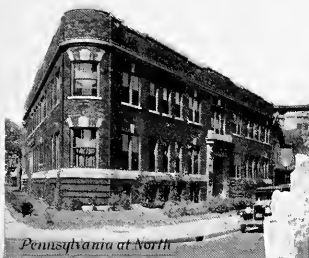
Pennsylvania at North
