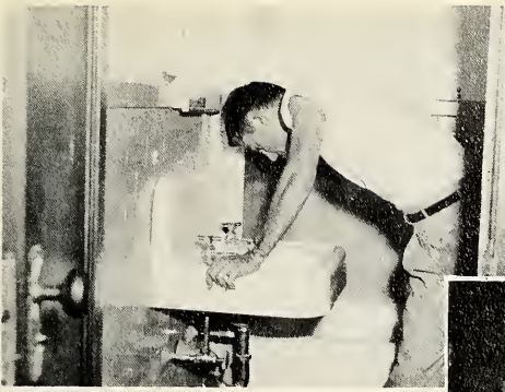
(Left)—Bill Price surveys the ever-present problem of a stopped up sink drain.
