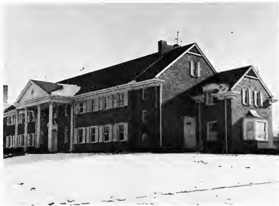
The Sigma Chi house is one of the largest fraternity houses on campus.
