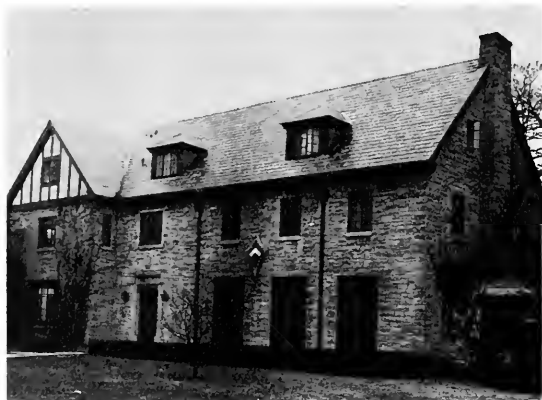
The ivy-covered Theta house awaits a brand-new addition.
