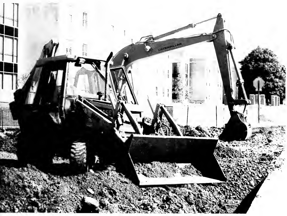
"Watch your step!" Many Butler students had to leave earlier for classes in order to make it on time. The mall was blocked off for several weeks while the heavy machinery went to work.
