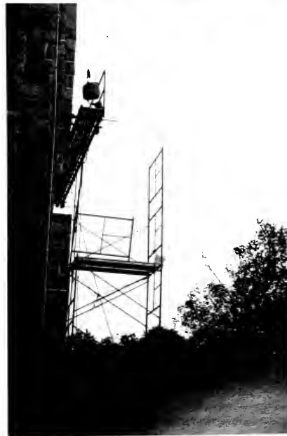
Above: Renovations of the outside of Jordan Hall took place all year long. Several classes had to move to different sections of the building to escape the high level of noise from the machinery.
