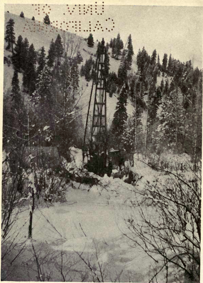
Work continues in spite of snow
