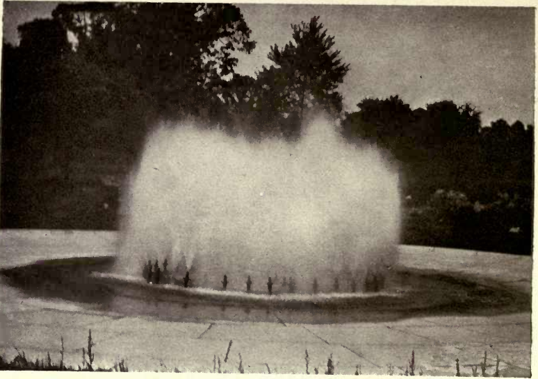
FIG. 67.—Aerator at Rye Pond. Borough of the Bronx, New York City.
