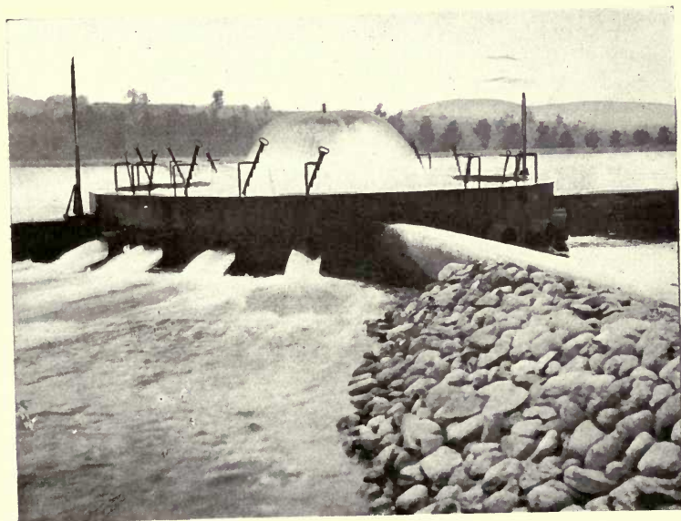
FIG. 66.—Aerator at the Ludlow Filter, Springfield, Mass.
