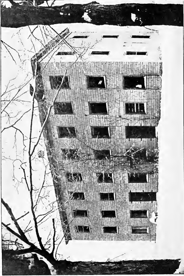
THIS IS THE LEAST RUINED OF THE THREE REMAINING BUILDINGS OF FAIRFIELD, AND IS THE LABORATORY SO OFTEN MENTIONED
